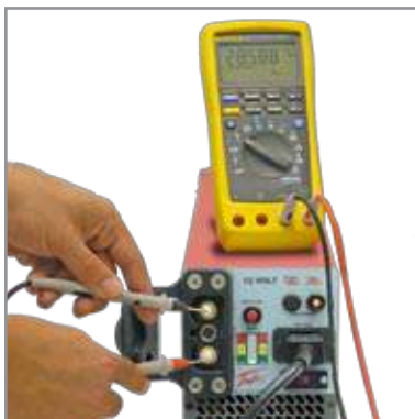
Figure 3.8.2 – Testing DC Receptacle
