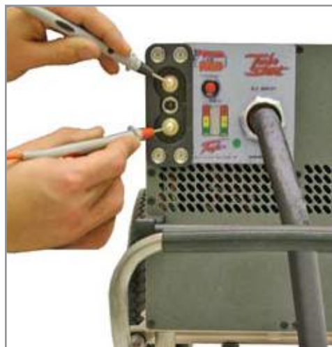
Figure 3.8.3 – Testing DC Receptacle
