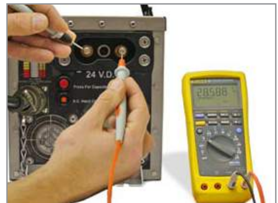
Figure 3.9.3 – Testing DC Receptacle
