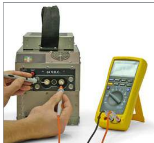
Figure 3.9.3 – Testing DC Receptacle
