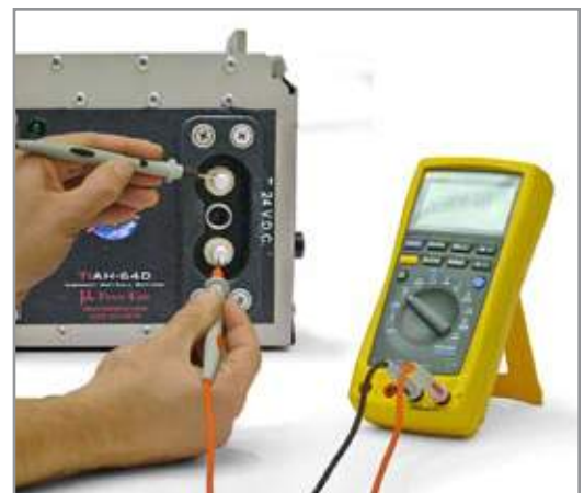
Figure 5.2.3 – Testing DC Receptacle
