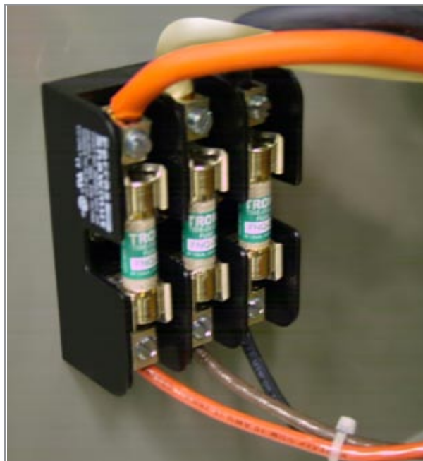
Figure 4.4.1 Replaceable Fuses
