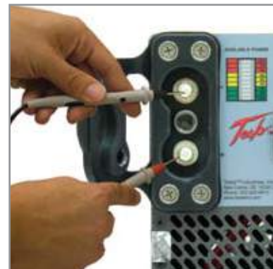
Figure 3.5.3 – Testing DC Receptacle
